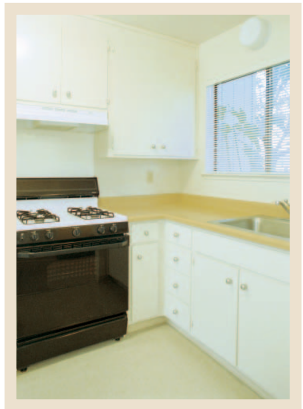
New appliances were installed at the Portola complex in Live Oak.
