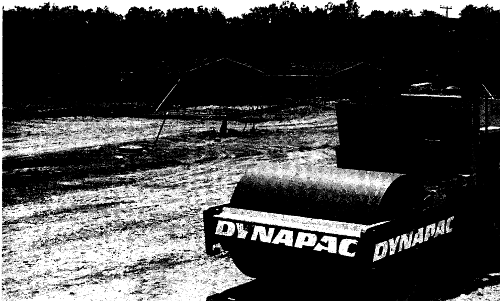
NEW MIGRANT UNITS: Construction is proceeding on schedule for 12 new housing units at Buena Vista Migrant Center near Watsonville. The units are expected to be ready for occupancy when the center opens for the summer of 1998.
