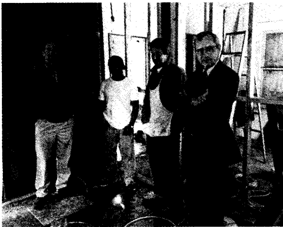
FIXER-UPPER: Extensive work is being done to get 113 Kaye Street in the Beach Flats area of Santa Cruz ready for sale. Norm Daly (far left) and Gene Arner (far right) of the City of Santa Cruz check the progress being made by contractor Luc DeFaymoreau and his assistant Anthony Garcia.
